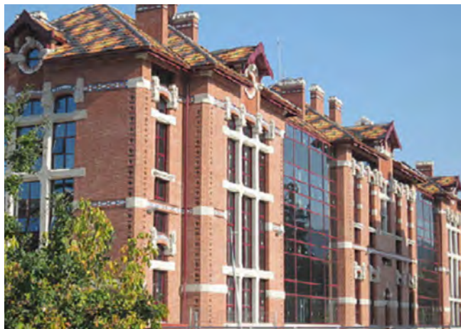
Basurto North Hospital, Bilbao, Spain
