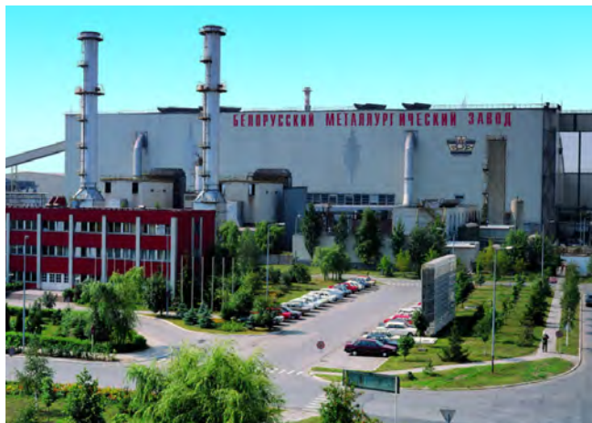
BMZ Steel Work, Gomel, Belarus
