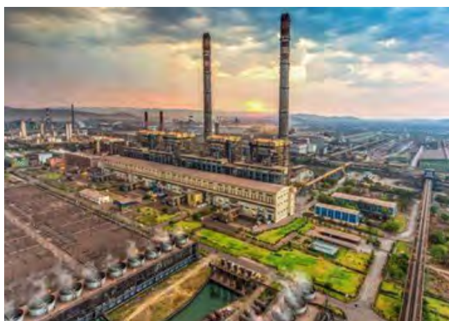
JSW steel, Mumbai, India
