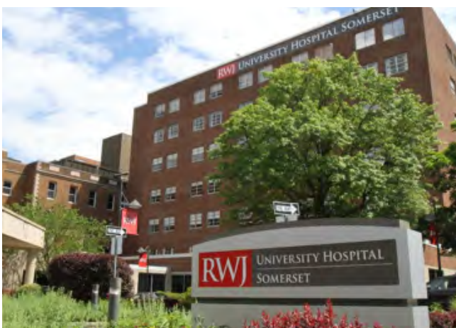
RWJ University Hospital Somerset, New Jersey, USA
