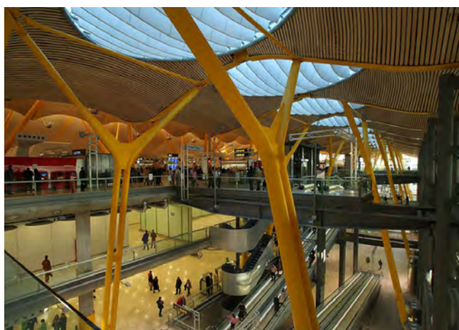
Madrid Airport, Spain
