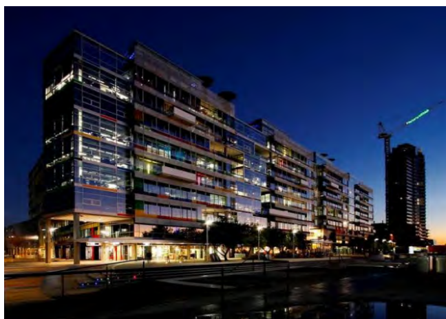
National Australia Bank, Melbourne, Australia
